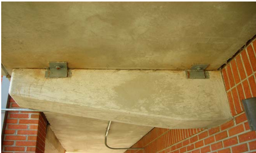
PHOTO #5, Building 4310 Failed beam, right side.
